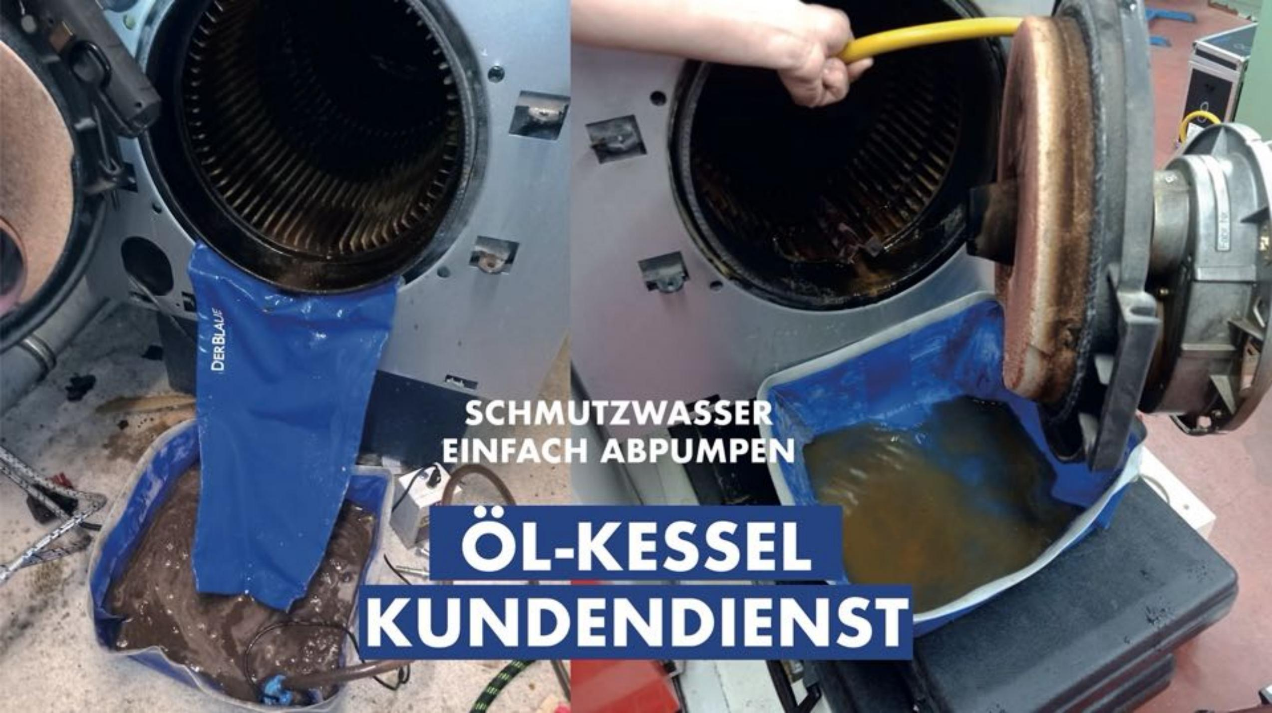
A person is shown using a yellow pump hose to drain dirty, brownish water from a boiler into a blue collection bag. The boiler is open, revealing a dark interior with a large circular grate. The blue bag is placed on the floor and is partially filled with the drained water. The text 'DER BLAUJE' is visible on the side of the bag. The scene is set in a workshop or industrial environment.
